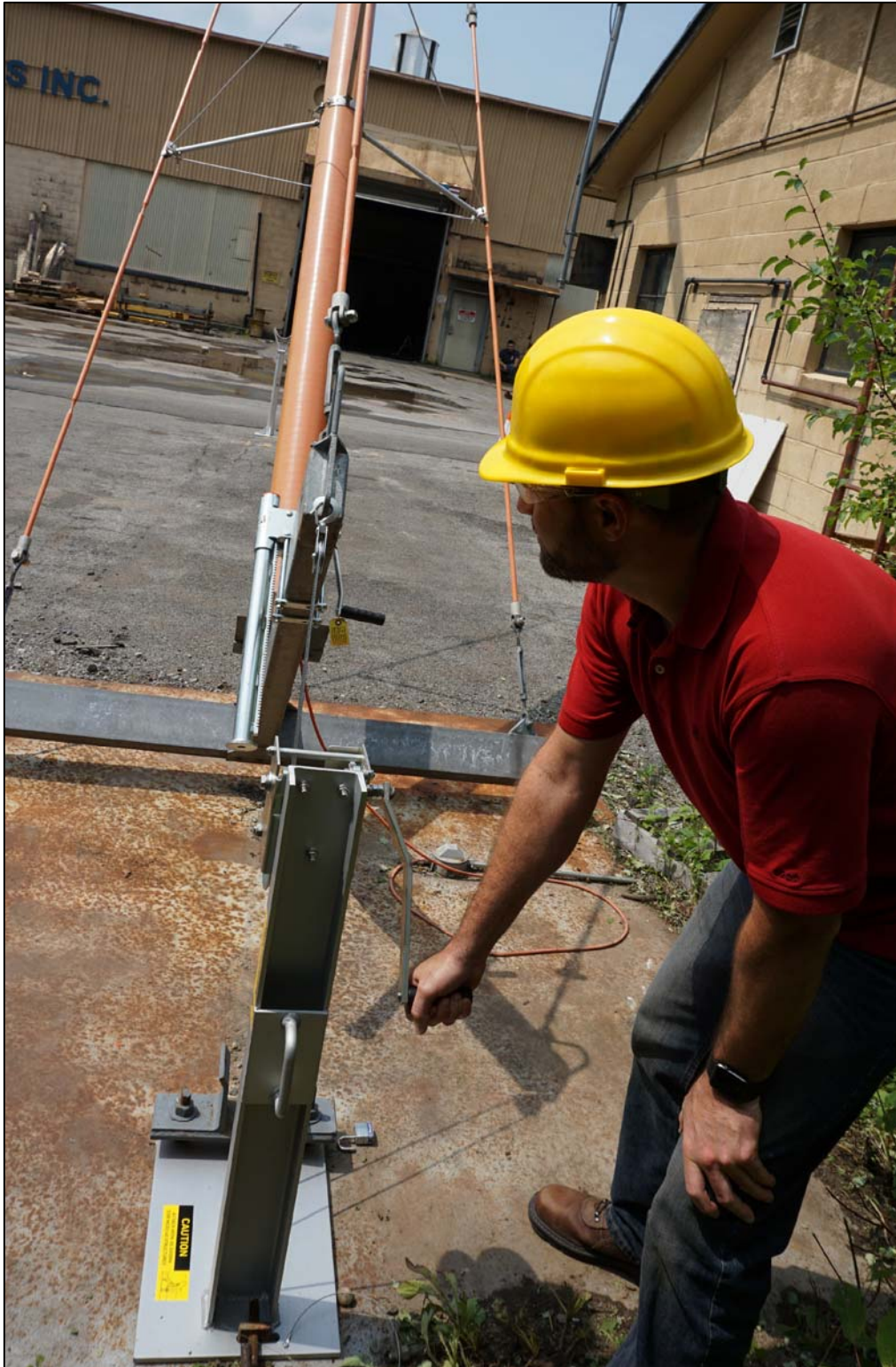
FIGURE 3-6 LOWERING MG-30/40 STRUCTURE (Ref. Section 3.3)
