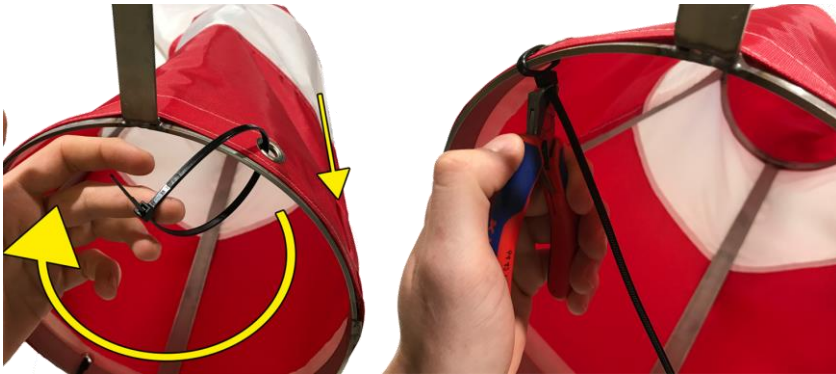
Image 1; Attaching the windsock
