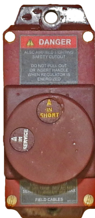
Figure 7: SCO - Series Circuit Cutout, ALSC
