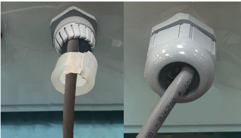
Figure 9. Passing Cables through the Conduit
