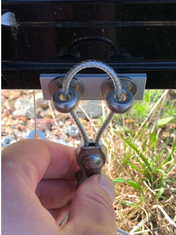
Figure 15: Mount washers and eye bolts
