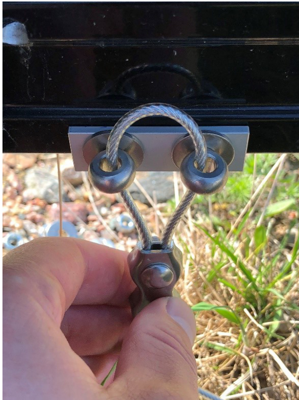
Figure 12: Mount washers and eye bolts
