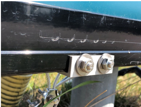
Figure 11: Mount washers and lock nuts
