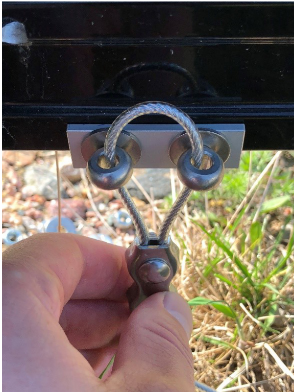
Figure 15: Mount washers and eye bolts
