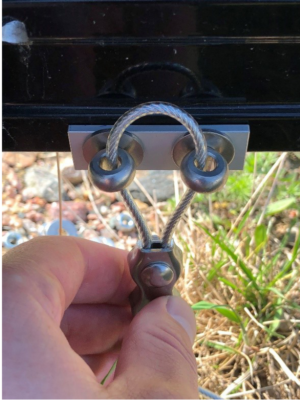
Figure 10: Mount washers and eye bolts
