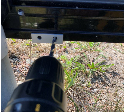
Figure 14: Drill holes through the profile
