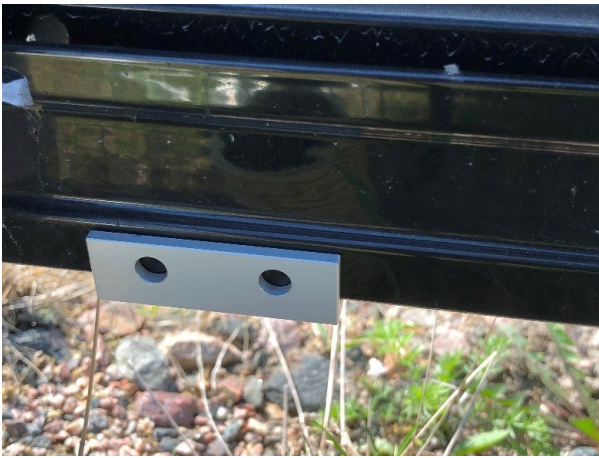
Figure 9: Place the bracket
