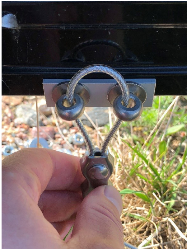
Figure 15: Mount washers and eye bolts
