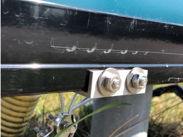
Figure 16: Attach washers and tighten lock nuts
