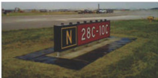
Strip Matting around a directional sign.
