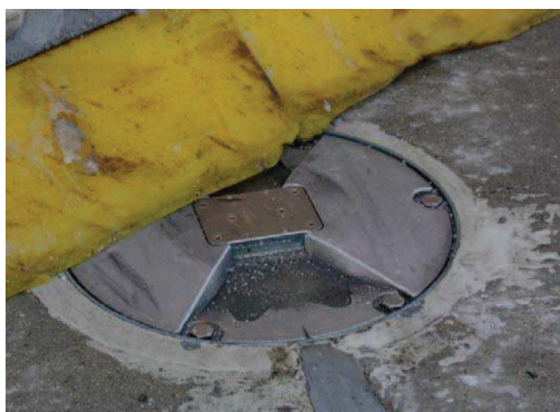
Figure 66: Snowplow blade with wear and steps between segments
