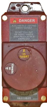
**Note** SCO - Series Circuit Cutout (1475.92.030) includes a micro-switch to detect removal of the SCO handle. The handle can be locked in position and can be placed in the Maintenance or the Test positions, which ground the CCR output and the field cable. Please refer to SCO Cutout manual 96A0294 for more details.
