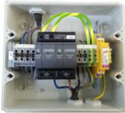
Figure 10: Overvoltage protection unit for the power and data cables
