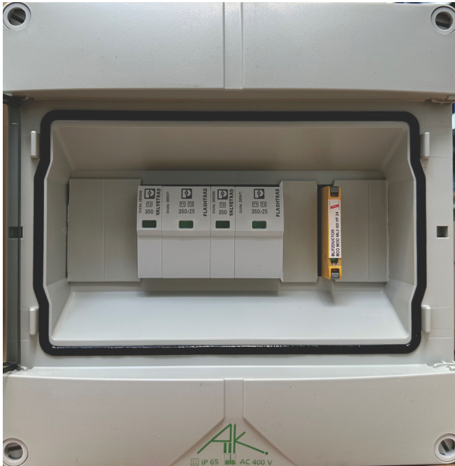
Figure 10: OLP Unit Surge Protection Devices
