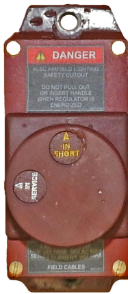
Figure 5: SCO - Series Circuit Cutout, ALSC
