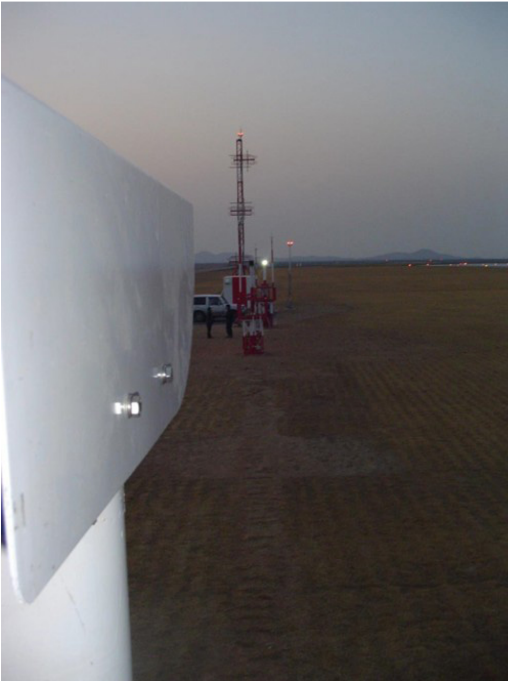
Figure 34. Mechanical Alignment Check
