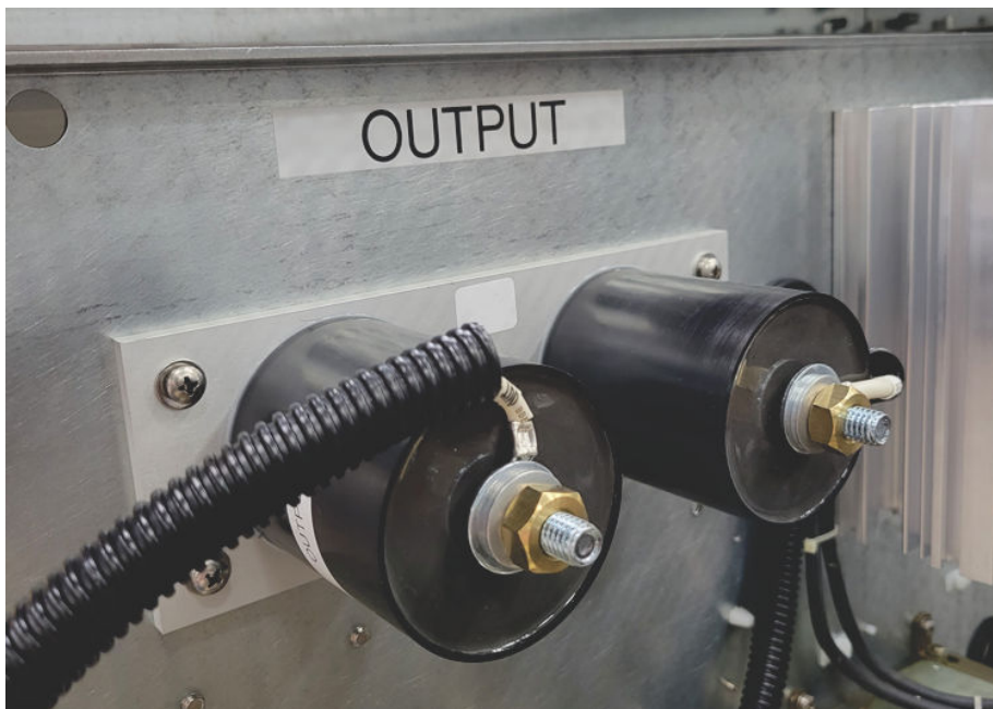
Figure 49: Output Lightning Arrestors
