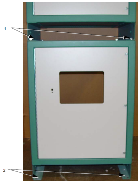
Figure 10: Location of Bolts for Stacking CCRs
