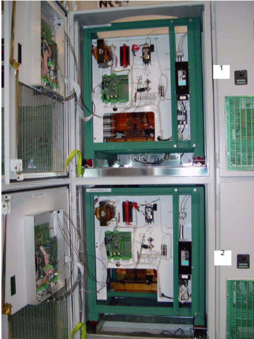
Figure 12: Powerpack Installation in SGRS
