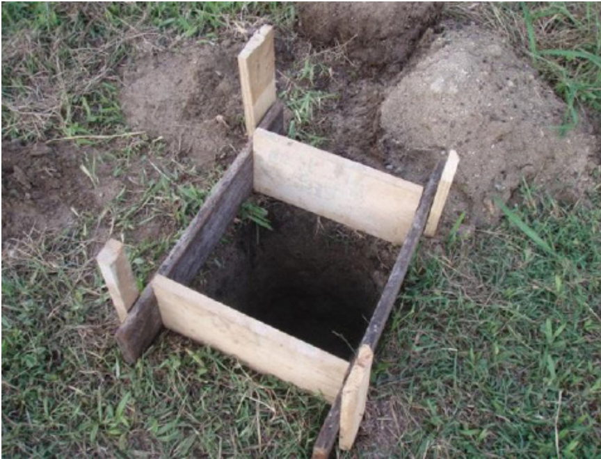
Figure 14. Foundation Hole with Form
