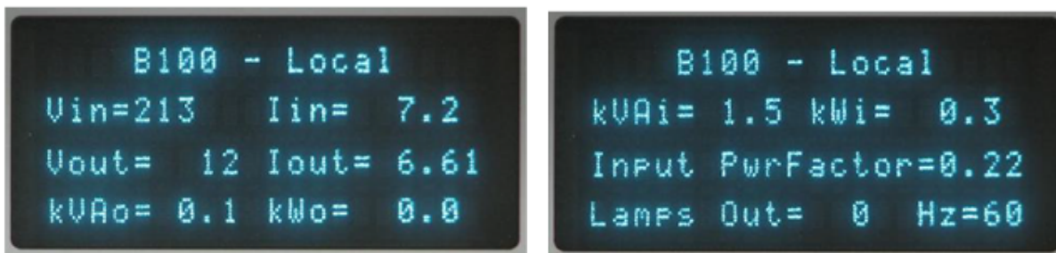
Figure 12: Displays - Additional Data Shown By Scrolling Down
