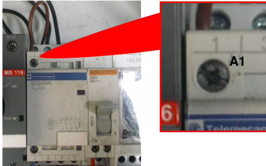
Fig. 8.- Locate pin A1 on the pump's relay.
