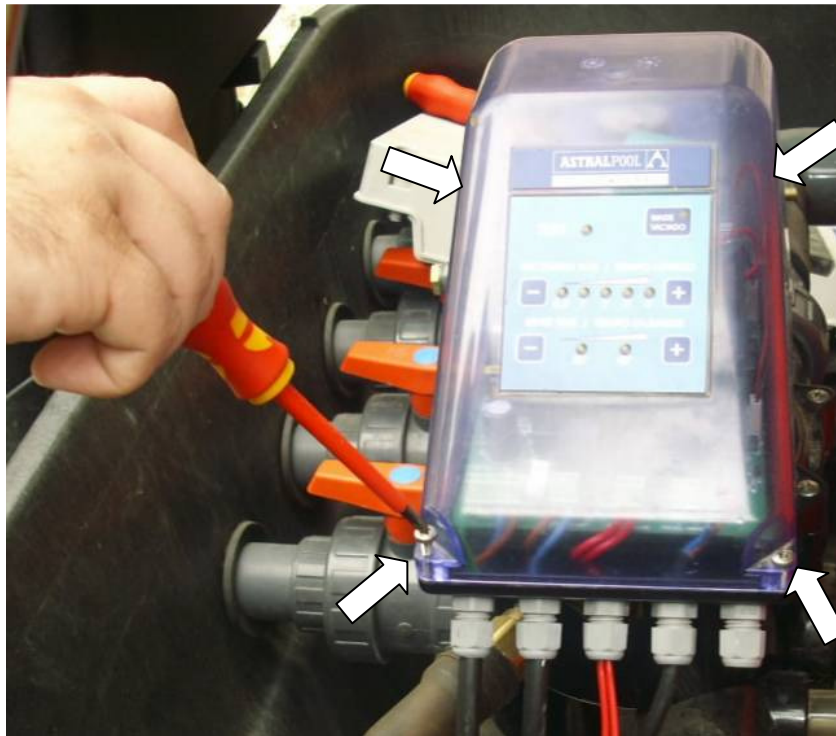
Fig. 1.- Unscrew the 4 bolts that fix the cover
