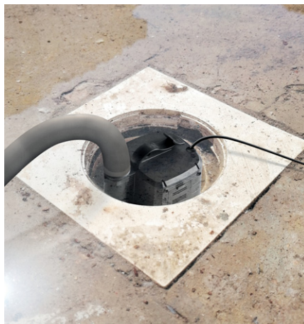
Sump pit installation Dauerinstallation in Brunnen
