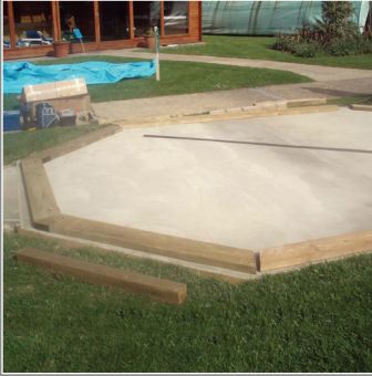
Concrete level base
