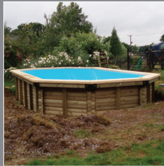
When constructed, install the liner and landscape the garden
