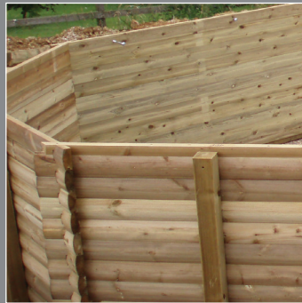
Build the wooden surround
