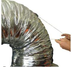
8 Run the cable around the duct and position the plastic duct so that it protects the blowing duct.
