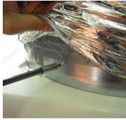
6 Position the duct on the frame and secure it using the 4 self-boring screws provided (there are holes in the duct framework).
