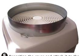
**S** Reposition the cover and attach it to the frame on the heat pump using the 4 long screws and washers provided.
