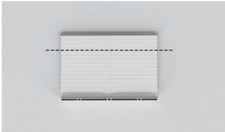
On a protected surface, carefully cut the vent at the desired location.
