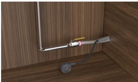
Briefly turn on the water supply and check for leaks, once you are satisfied the connections will not leak turn off the water supply.
