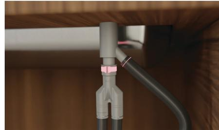
Thread wire clip on to the hose before fitting hose to the supplied hose joiner. Secure using the hose clamps. Fit to the Air Gap Kit. Ensure hose is routed straight to the joiner, remove any excess drain hose.
