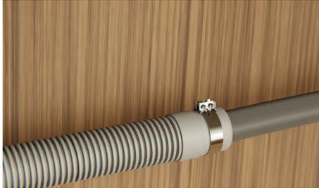
Pull the hose through the drain hose support before threading the hose clamp onto the hose and fitting to the sink trap. Secure to trap using the clamp. Ensure hose is routed straight to the trap. Unplug or drill out the waste tee before securing joiner to sink trap or waste tee.
