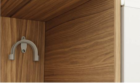
Install the drain hose support to the back wall, as close to the underside of the countertop as possible. Refer to 'Plumbing & electrical considerations' for minimum install heights.
