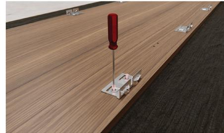
Secure the side brackets using two screws per bracket. Ensure side brackets are fitted tightly and the fasteners are secured straight.
