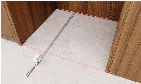
Measure the depth range of the alcove ensuring the minimum depth range has been met.
