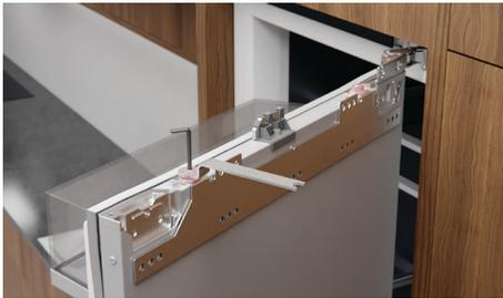
Remove both washers and nuts and set aside. Lift the panel brackets upwards to remove.
