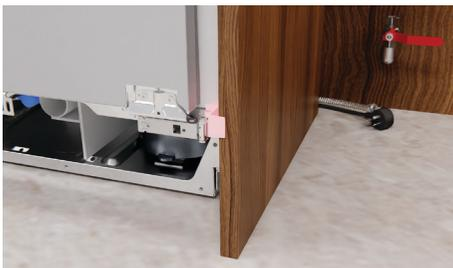
Push product into alcove while pulling the hose and power cord. Ensure the gauges touch the alcove end, the hose doesn't kink and the power cord remains free and untangled.
