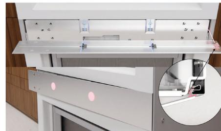
Ensure the 2x centre clips are on its marks and the side hooking clip on place.
