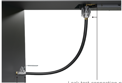
Leak test connection points
