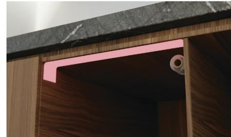
Align the supplied moisture protection tape to the cabinetry as shown.
