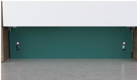
Ensure door swing is unobstructed before securing the sound seal sheets to the metal toe kick plate using the supplied double sided tape.
