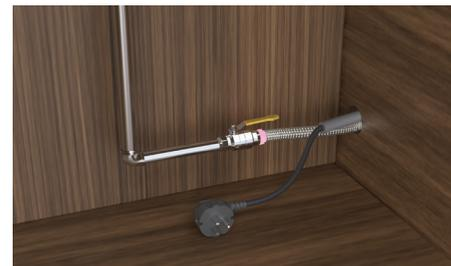
Briefly turn on the water supply and check for leaks, once you are satisfied the connections will not leak turn off the water supply.
