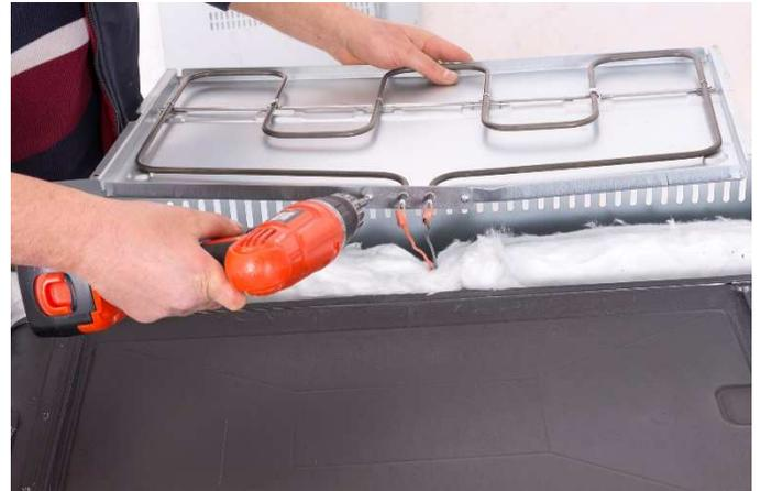
Remove screws with the help of screwdriver and remove cables on the heating element. Push from sides of heating element cover plate and pull towards back side of oven as shown in picture.
