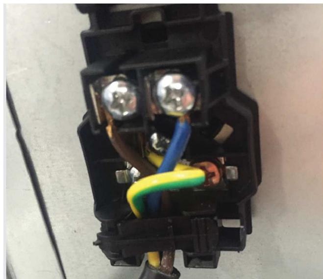
The mains cord connection on all the appliance where small terminal box is used must be made as shown in the image.
