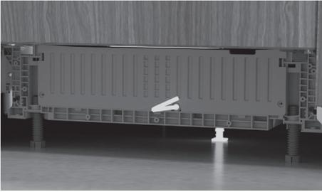
If needed, adjust the Dishwasher within the cavity before tightly securing in place.
