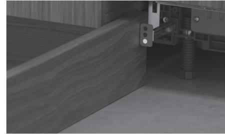
Mark the pilot hole locations for each bracket. Measure the centre of the panel and mark 237mm to each side. To determine the height of the brackets, measure the height of the lowest bracket hole against the toe kick panel.
