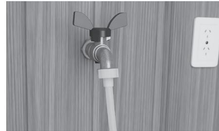
Ensure the rubber washer is fitted when connecting the inlet hose to the tap. Hand-tighten into place. Using a spanner or pliers, turn a further 180° to secure. Avoiding over-tightening. Do not turn water supply on. The Dishwasher must be powered on for the flood protection feature to be enabled.
