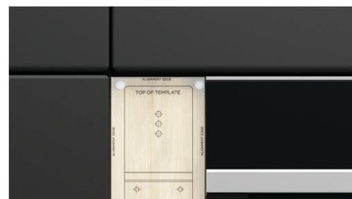
Ensure the template is completely flush against the cabinet and all four corners are secure.
