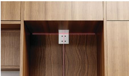
Measure the height from floor to the front overhang and mark on rear wall.
