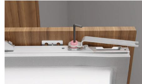
Loosely tighten the side screws and the top M8 washers using the spanner and L key provided in the install kit.
