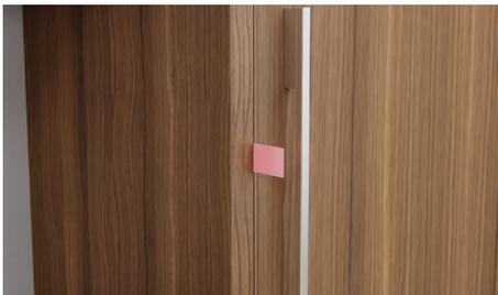
Using a piece of tape, fit a tab on the door to assist in opening the door without disturbing panel settings.
