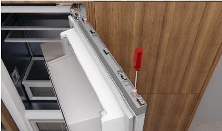
Remove the top cover using a powered driver. Set aside.
