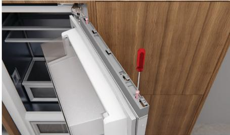
Remove the top cover using a powered driver. Set aside.
