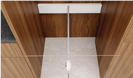
If required, install a spacer at the rear of the cavity to bring depth to 600mm.
