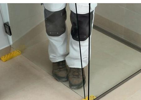
Place the shower door in the support so the two hinges sit tight against the tiles. Then check that the shower door is positioned correctly with the right clearance on all four sides. Up, down and sideways. When the two steel hinges have been screwed to the wall, the shower door can be adjusted by +/- 2-3 mm in all four directions.
