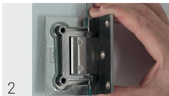
Fit the two stainless steel hinges to the shower door in the mid-position in the cut-out in the glass.
