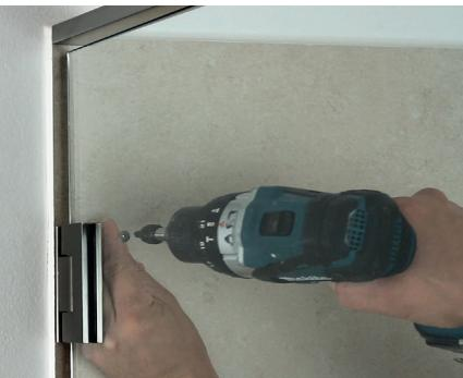
Place the shower door on the support again and screw into place with the six screws provided.
