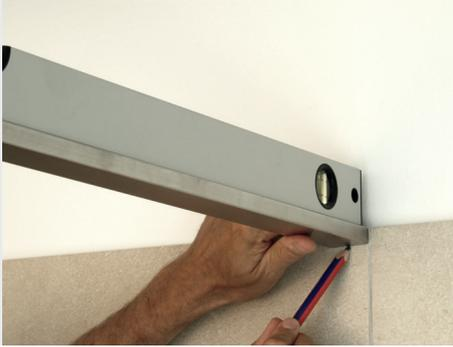
Hold the top rail horizontally using a spirit level and mark the tiles around the top rail.
