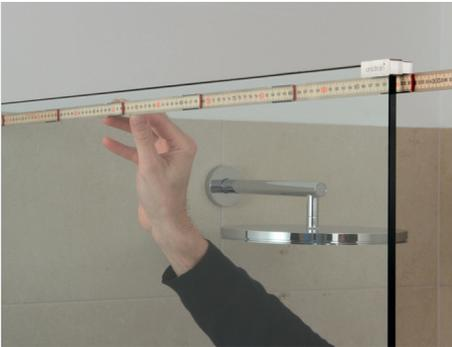
Measure the depth of the shower cubicle from the tiles on the wall to the unidrain® glass bracket.
