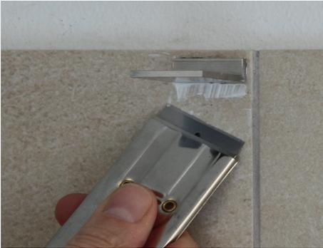
When the foam block is removed, there may be some excess glue residue that must be removed with a scraper or a utility knife.
