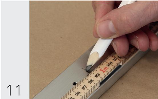
Mark the measurement on the top rail.
