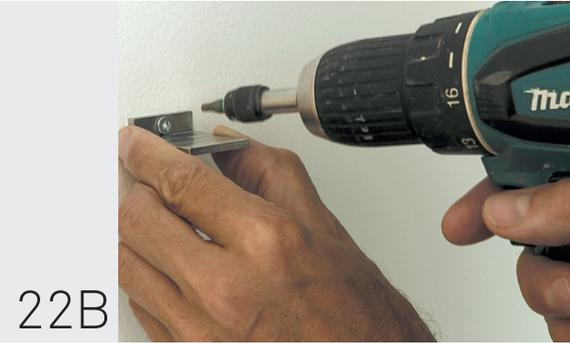
It is possible to screw the wall bracket in place if desired. If the top rail is installed on a wall surface to which the glue cannot stick, such as painted surfaces, using screws is required.
