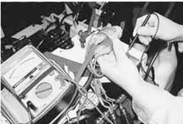
2. Check if battery voltage is applied to the 50 terminal in starter switch ON position.
