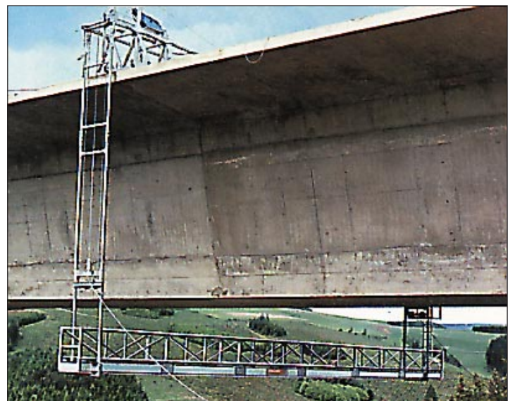
Fig. 4 - Operation of suspended platforms for the inspection and maintenance of bridges (TU-32H).
