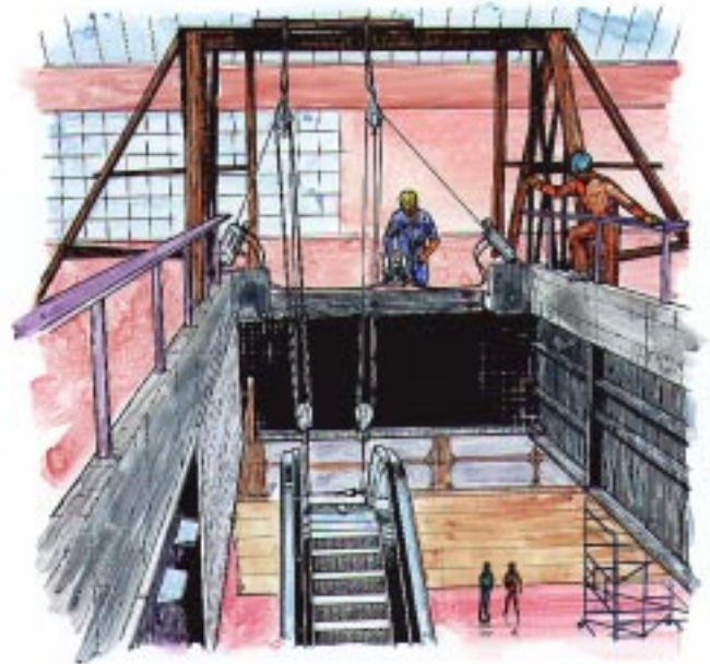
Fig. 27 - Installation of mechanical escalator (TU-16H)
