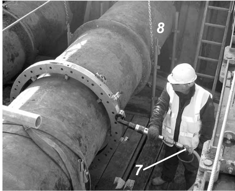
Figure 2-2. Potential operating hazards of the LCSF. See the descriptions below.
