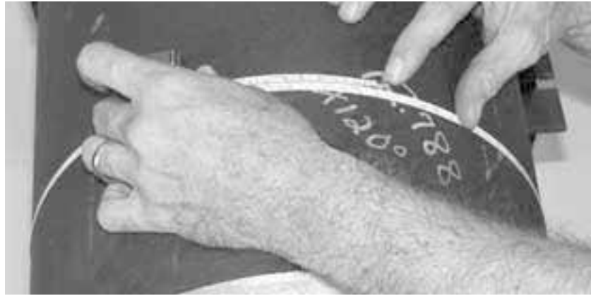
Figure 5-3. Verify the pipe circumference by measuring.
