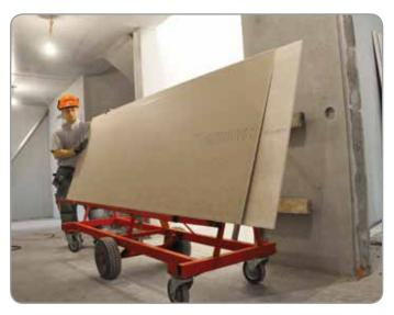
The Transit Bench as a stable workbench to enable easy and precise cutting of plasterboard.
