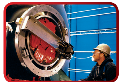
LCSF with bridge slide accessory shown on Steam Generator during replacement
