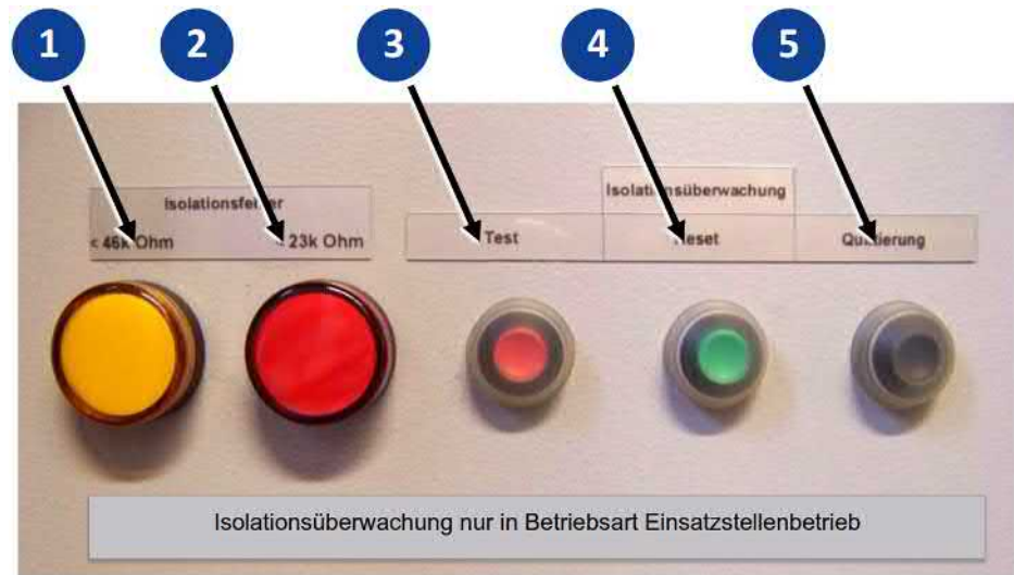
Fig. 8-6 Insulation monitoring
