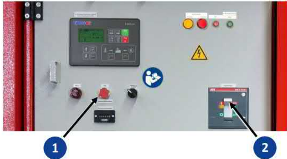
Fig. 7-5 Differential current release
