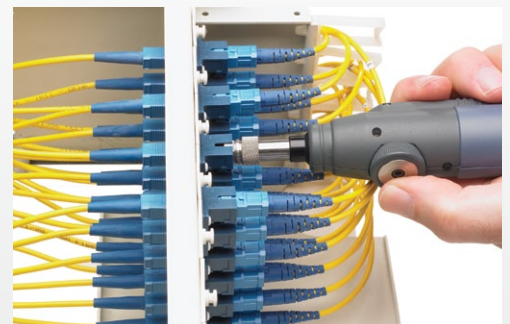
Patch panel bulkhead inspection
