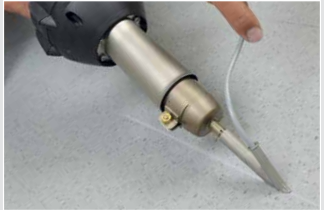
Plastic and linoleum floors
