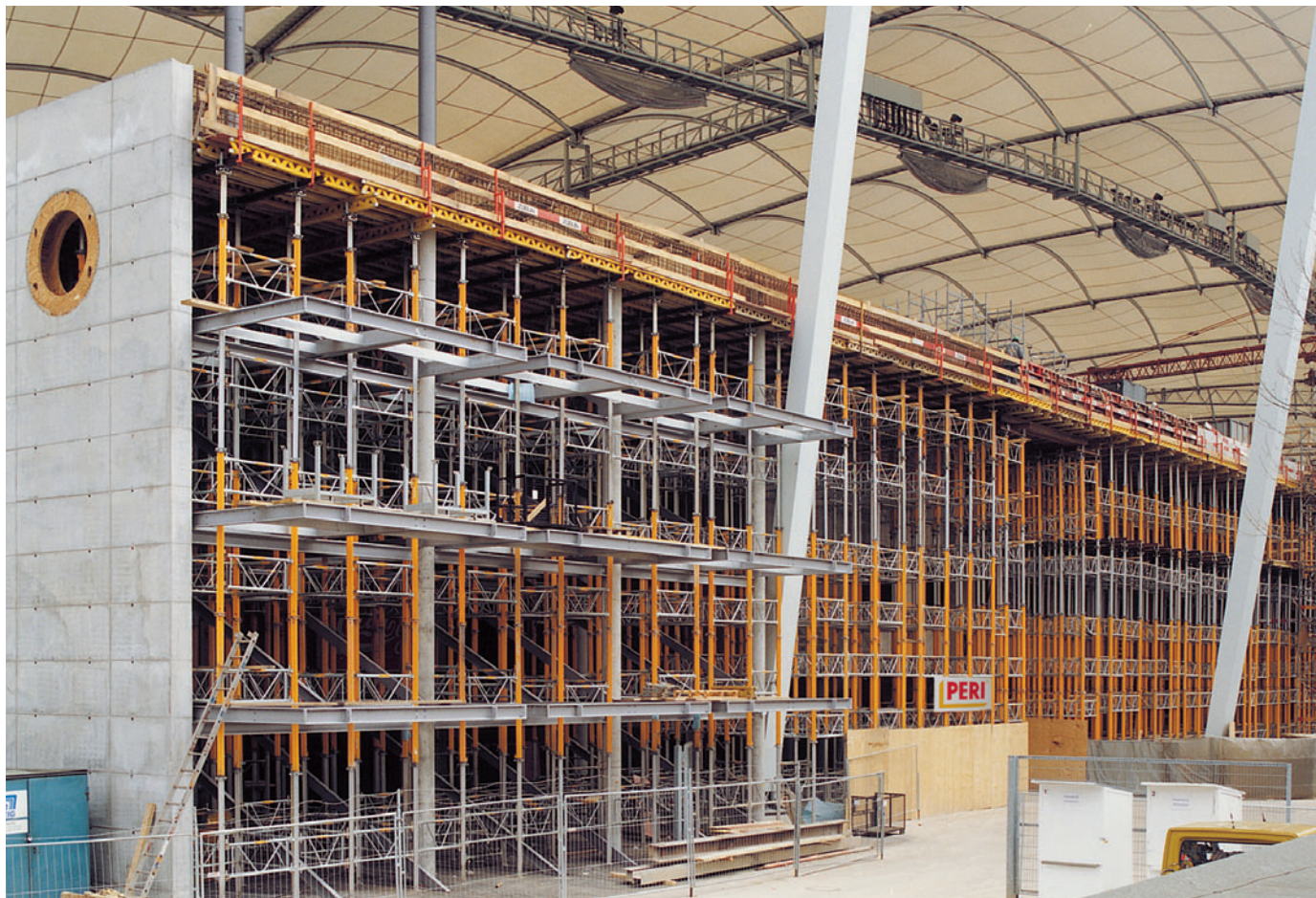
14.00 m high MULTIPROP falsework over an area of 3500 m 2 .
