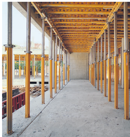
MULTIPROP 350 with MULTIFLEX slab formwork.
