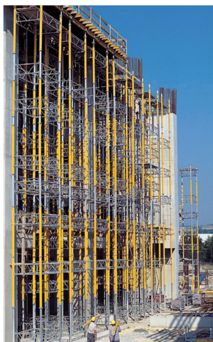
20 m high MULTIPROP towers supporting a cantilevered slab.
