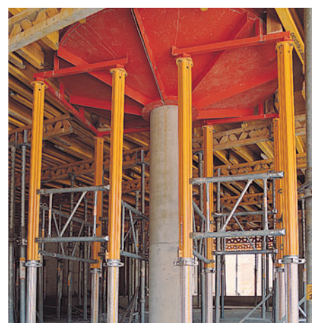
MP 350 with frames supporting column capital formwork.
