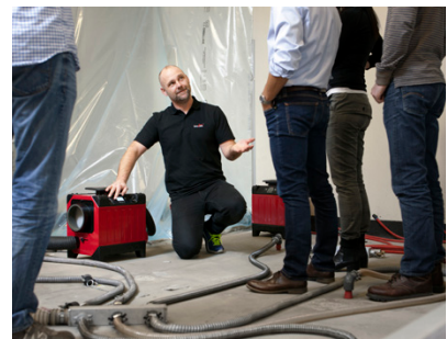
Practical tests of different drying techniques are carried out at our seminars. In our own building laboratories, theory and practice are combined; water damage in different structures is dried and evaluated with measurements.
