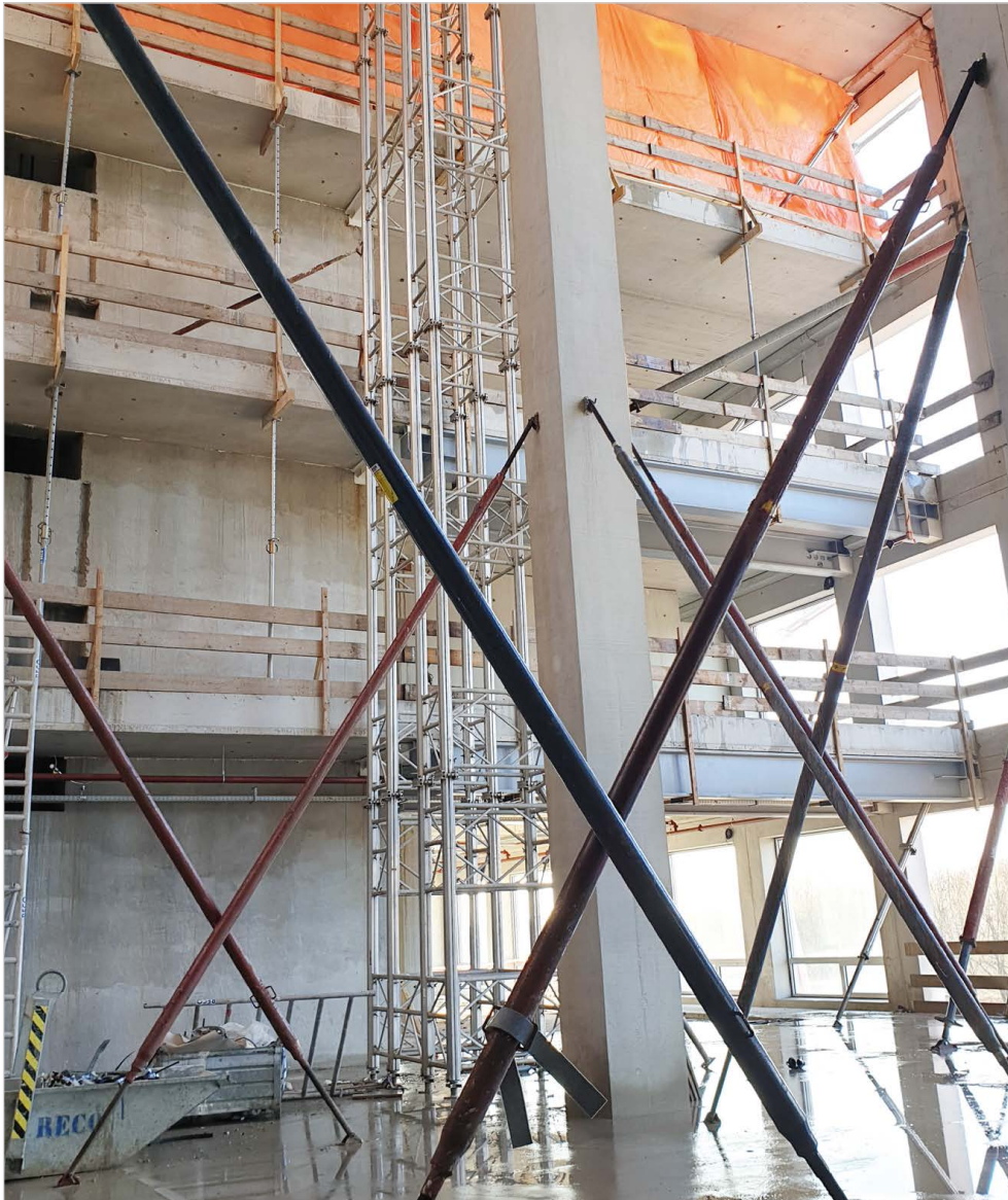
Precast concrete elements aligned and supported with TITAN RSK push-pull props (size 8 shown here) up to a height of 7.60 m
