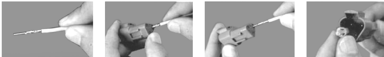
Figure 7-12. DT/DTP Contact Installation
