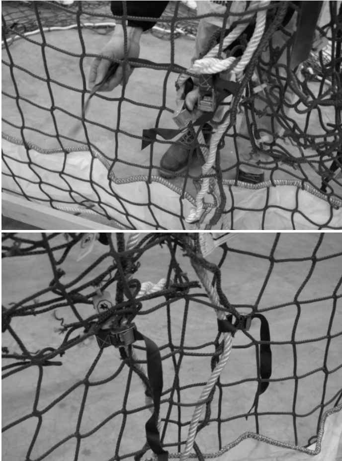
Figure 16. Interconnecting rest of vertical net sides
