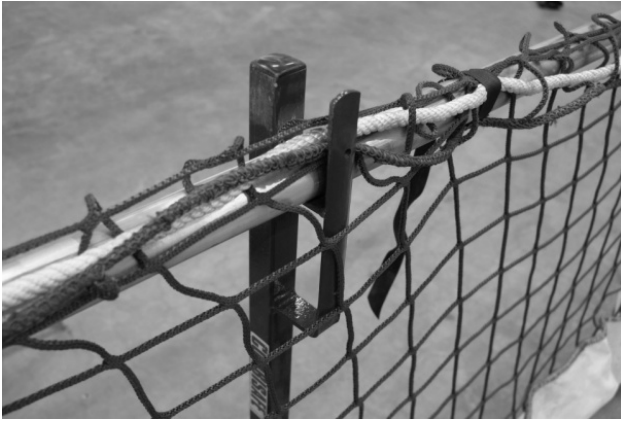
Figure 11. Net placed in the guard rail holder
