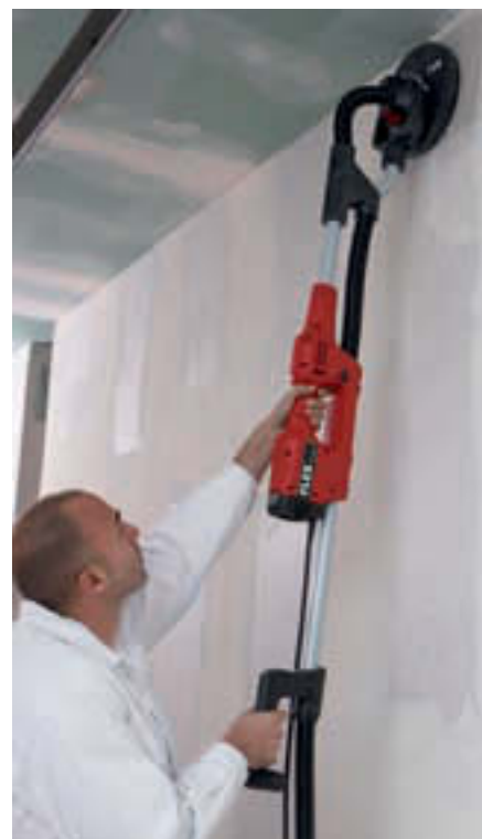
Quick and easy adjustment of the telescopic handle enables you to reach all heights in one process.
