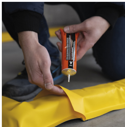
Attach corners using Type A Glue
